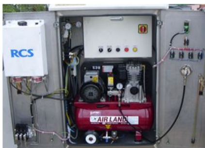
Fig. 3. Photo of rail coating system installed in Busan Metro Line 3.
