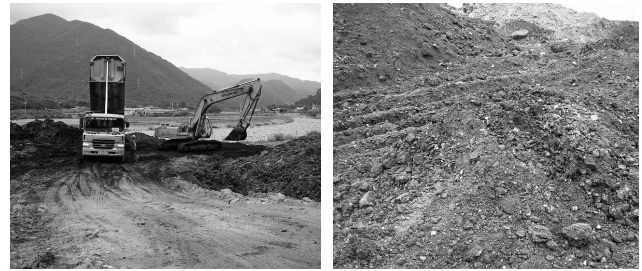
Fig. 7. Scene of recycling waste foundry sand as filling soil.
